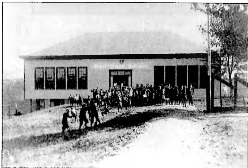
Merrimack School built 1914. Photo from Huntsville-Madison County Public Library Archives.
