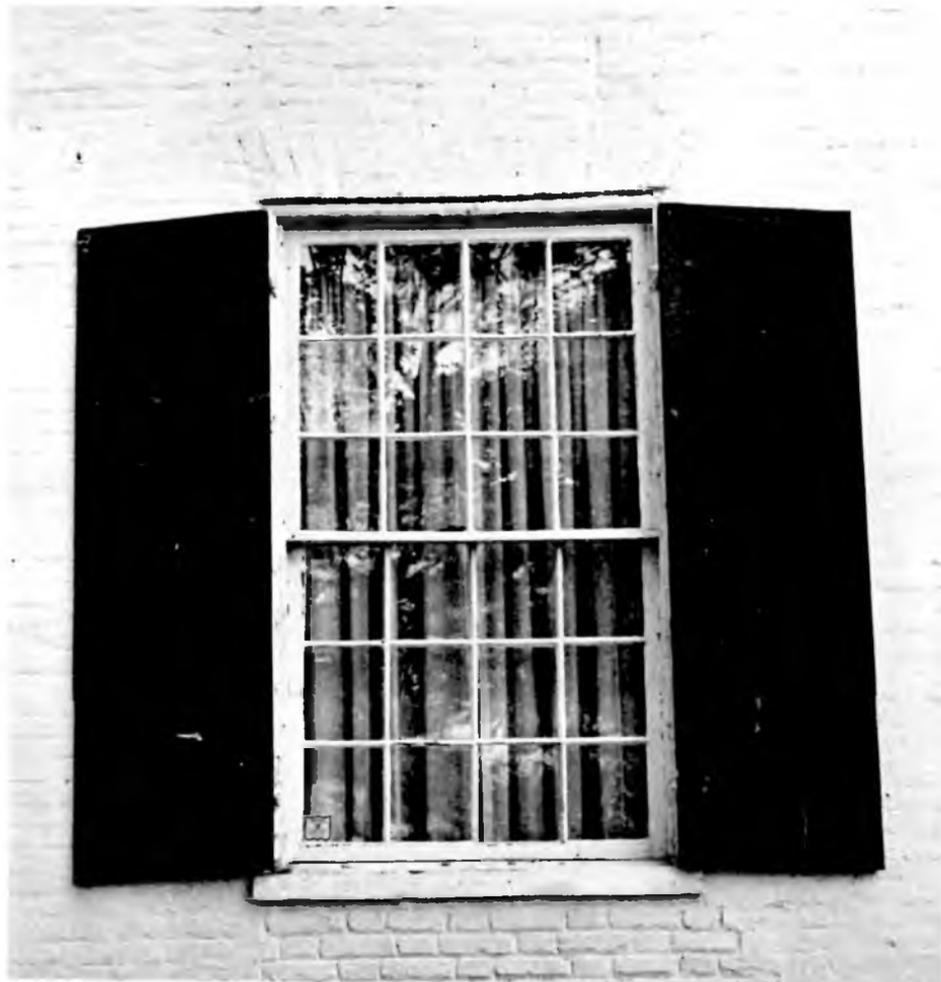
eral period houses. The window jambs (vertical wooden sides of a window) are semicircular on the outward edges--a frequent and elegant touch in Federal period architecture.
