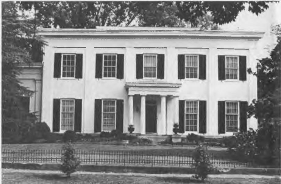
an exquisite Greek Revival design. It is a regular masonry block with pilasters employed to create the rhythm of a colonnade while an exceedingly low pitched roof makes the house appear to end at the cornice. A wide frieze spans the house above the pilasters. The windows are symmetrically spaced with the first floor ones extending to the floor, a common Greek Revival treatment. The porch is a miniature portico of four fluted Doric columns supporting a fully defined entablature.
