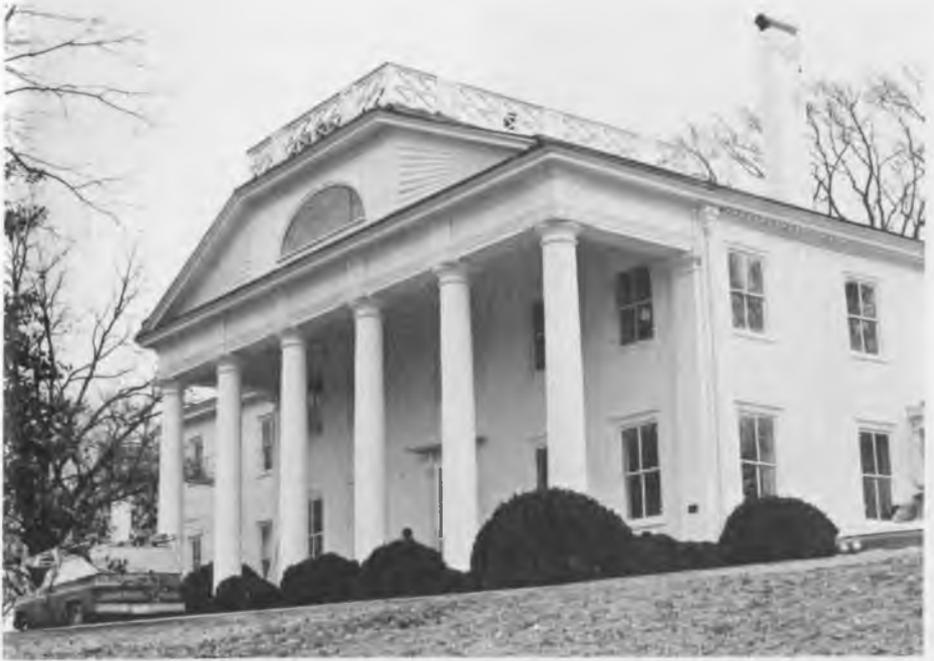
Steele had the task of fitting a giant portico onto a Federal house. Greek Revival was the current rage, but a two-story porch in that massive style would overwhelm the delicate detailing of the existing structure. The solution he chose was to erect a portico with the scale of the Greek Revival but lightened with Federally derived motifs. It features six colossal columns of the Roman Doric order which are unfluted and more elongated than the Greek and hence less massive.
