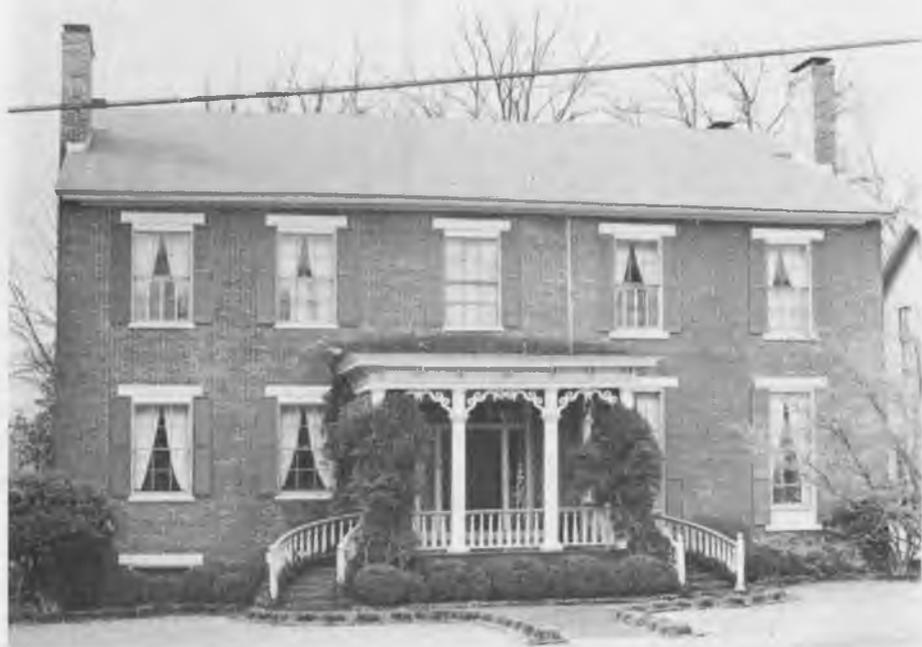
erected by Steele in 1826-7 is the south side which is in the Federal style. However by 1853-5 when Steele built the two northern bays, architectural tastes had altered. Although the addition appears to match the original, the windows indicate that a change has occurred; the first story windows are taller with paneling beneath, a hint that even greater changes might appear on the interior where, in fact, the parlors have marble Italianate mantles.
